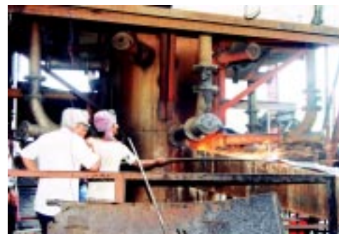
Divided blast cupola in a foundry
