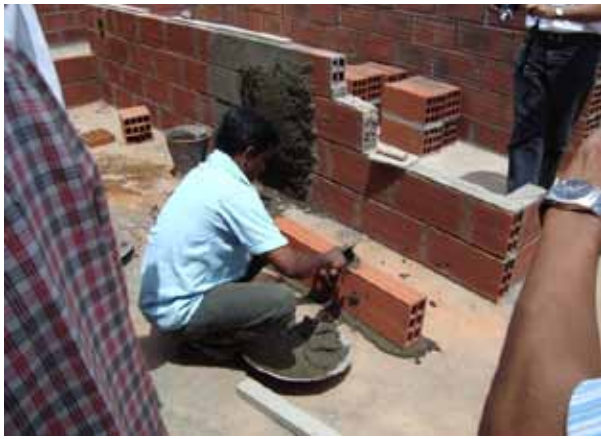
Demonstration of improved construction practices at Wienerberger plant
